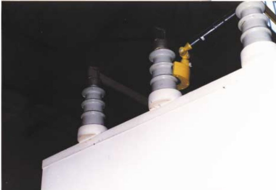
Figure 7: Cleaning of 30 kV busbar supports
