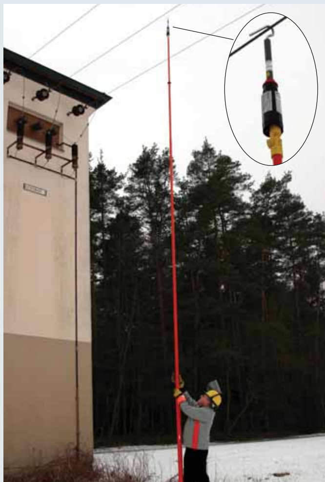
Telescopic rod for PHE III Test Head.
