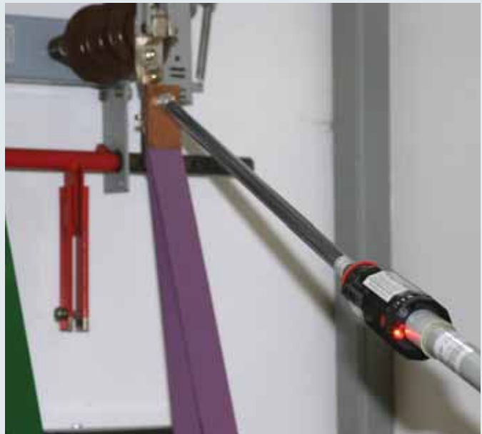
PHE III Voltage Detector with visual and acoustic indicator used for an indoor switchgear installation.
