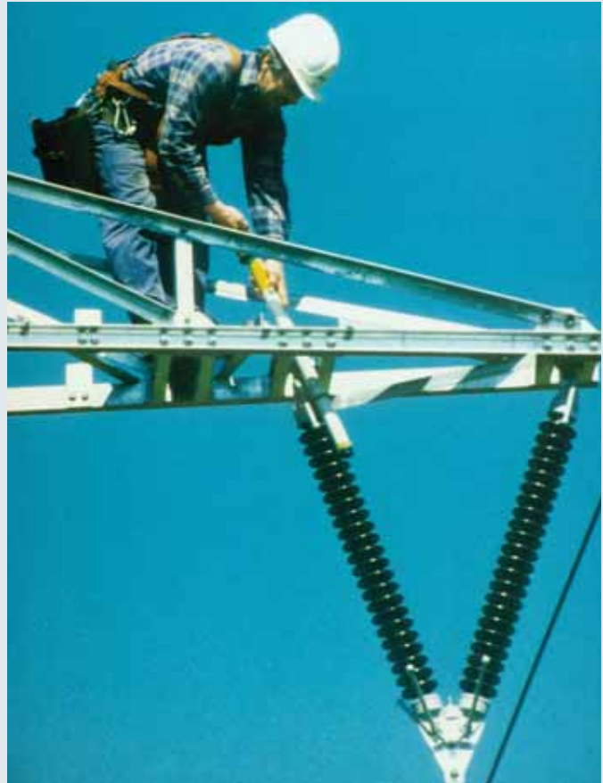
Distance voltage detector used for a 110 kV overhead line.
